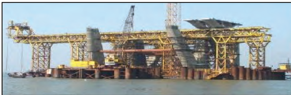
Figure 6.5: Erection of precast segments on scaffolding; all precast segments are lifted at one location by a lifting frame and slid on top of the scaffolding longitudinally
