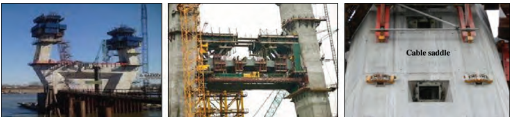
Figure 6.3: Upper pylon construction
