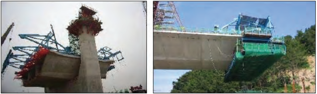
Figure 6.30: Form traveller erection arrangement
