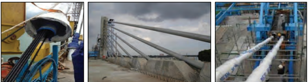
Figure 6.24: stay cable system
