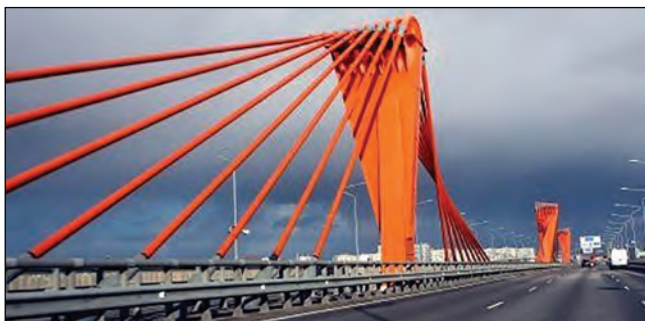
Figure 2.22: Pure fan cable arrangement – Riga Southern Bridge
