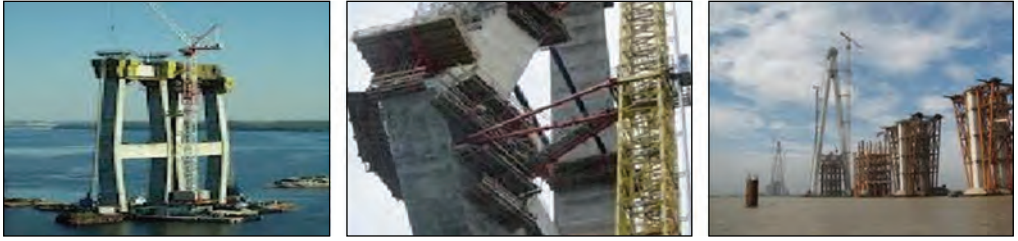
Figure 6.2: Tower crane for pylon construction
