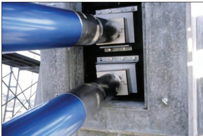
Figure 5.6: Odawara—shims at mast anchorage
