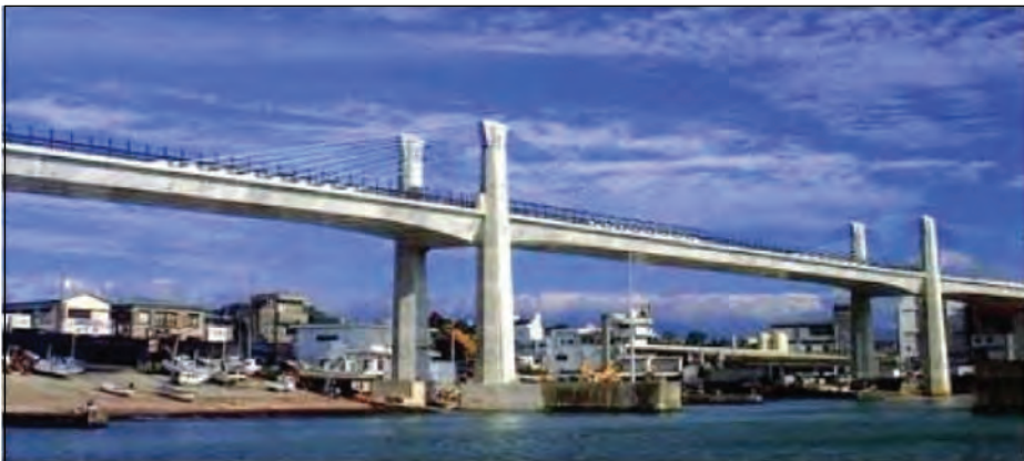
Figure 6.31: First Extradosed Bridge—Odawara Blueway Bridge.
