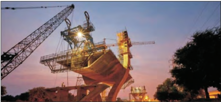
Figure 6.34: Bridge Builder arrangement on pylon-span
