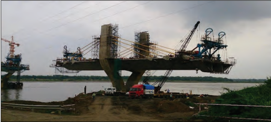
Figure 6.7: Balance cantilever technique
