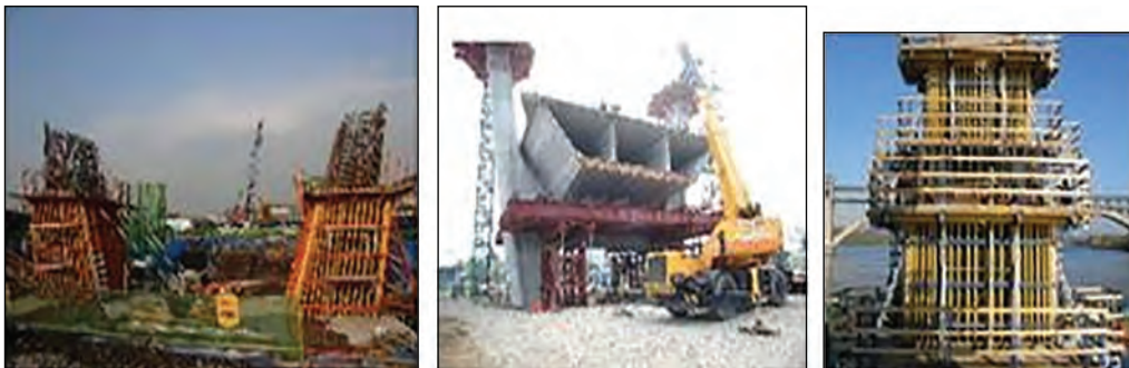
Figure 6.1: Pylon and pier-table casting
