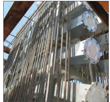
Figure 5.10: View of multitube saddles (copyrights: Freyssinet)
