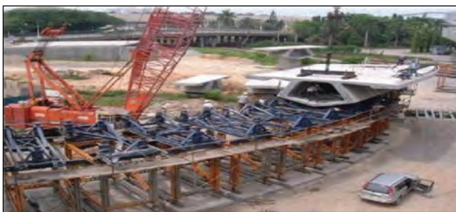
Figure 6.4: Erection of prefabricated segments on scaffolding
